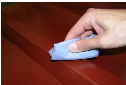
Figure 2: Cleaning the adherent surface
