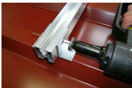
Illustration 18.1: Attaching the rivet depth gauge
