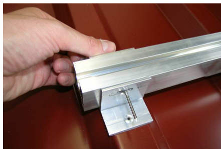
Illustration 17: Inserting the second dome head rivet
