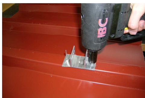
Illustration 10: Riveting with standard rivet head
