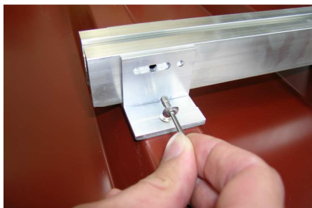
Illustration 16: Inserting the first dome head rivet
