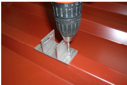
Illustration 5: Drilling through the roof surface
