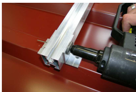
Illustration 18.2: Riveting with the rivet depth gauge
