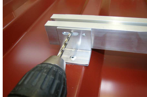
Illustration 12: Drilling the carrier rail
